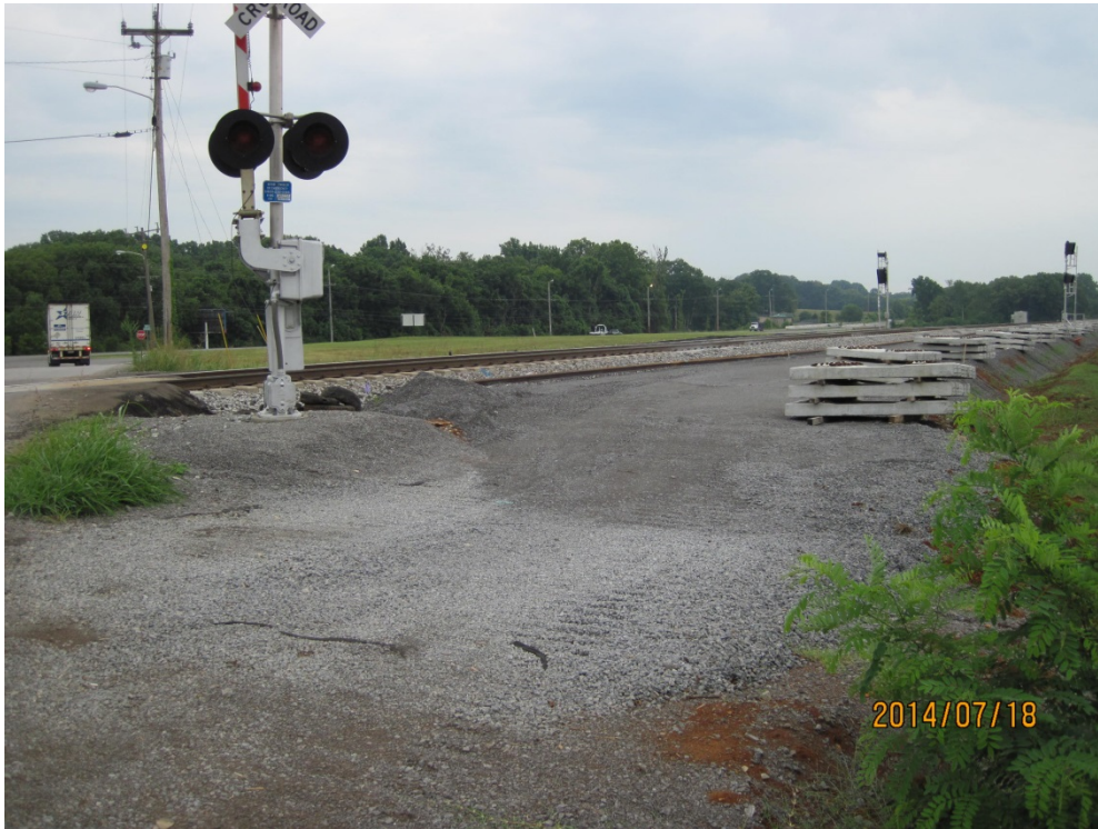
Photo 3: Railroad track facing south
