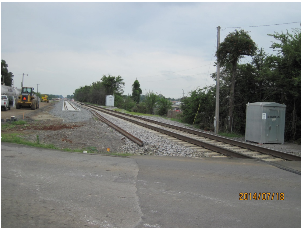
Photo 4: Railroad track facing north
